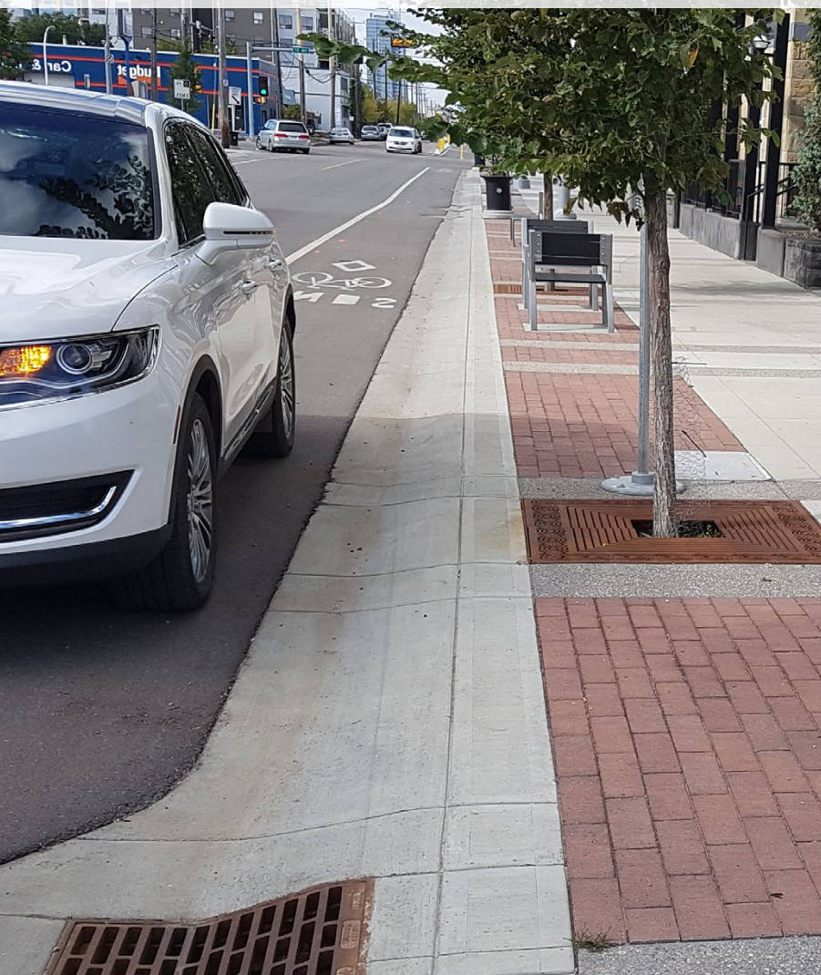
Stormwater run-off enters the tree vault via the catch basin, for treatment and flow
