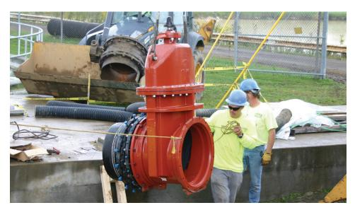
**AWWA C515** – The all ductile iron body, bonnet and seal plate resists corrosion and offers the same long service life as gray iron, but with less weight. It has increased strength, toughness and impact resistance. Each valve is pressure rated for 250 psi and tested for 500 psi performance which meets or exceeds AWWA C515.
