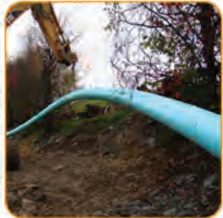
With PVC's proven long service life, Fusible Brute (CIOD) and Fusible Series (IPS) pipes are available in sizes ranging from 100mm (4") to 900mm (36") with larger sizes in development. The proprietary PVC formulation, fusion process as well as our licensing and training program allow for the consistent, reliable fusion of Fusible Brute and Fusible Series pipes to create piping systems of unparalleled strength.
