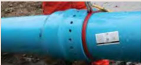
**3** One Ring at a time, place ring over pin holes and tap pins in until they bottom out on the inner groove.
