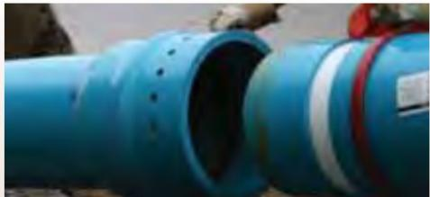
**2** Insert spigot up to the insertion line, aligning the internal ring and the pin holes.
