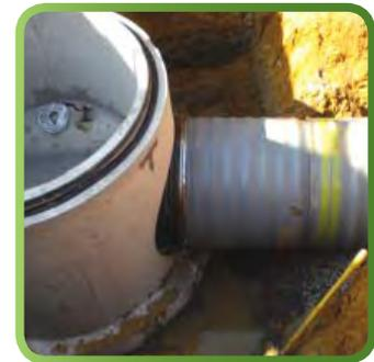
Boot Connection Directly to SaniTite HP
