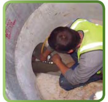
Typical ASTM F1417 Air Test
